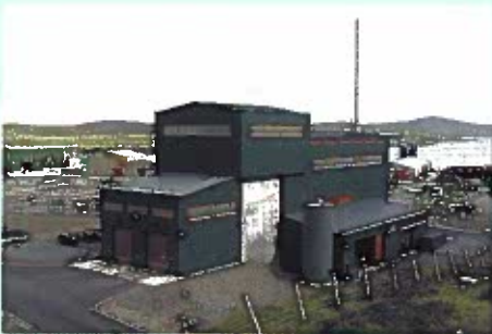
Energy Recovery Plant
